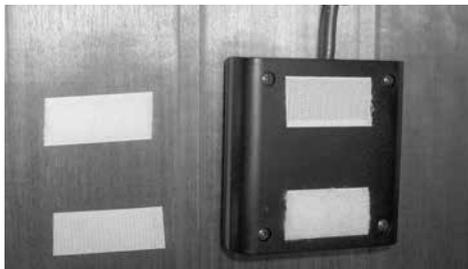
Then affix the button again and lead the connection line to the controls
